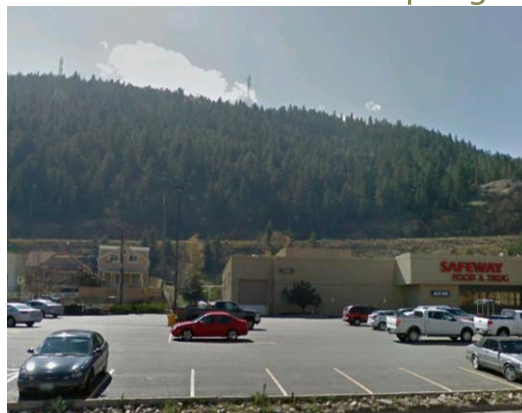
View of the eastern rock fall mitigation area from Colorado Boulevard, in front of Safeway
